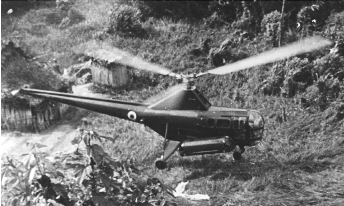
A Westland Dragonfly HC2 helicopter evacuating a casualty from a jungle clearing in Malaya. Powered by an Alvis Leonides air-cooled radial engine, the Dragonfly could lift three passengers or two stretcher cases.
