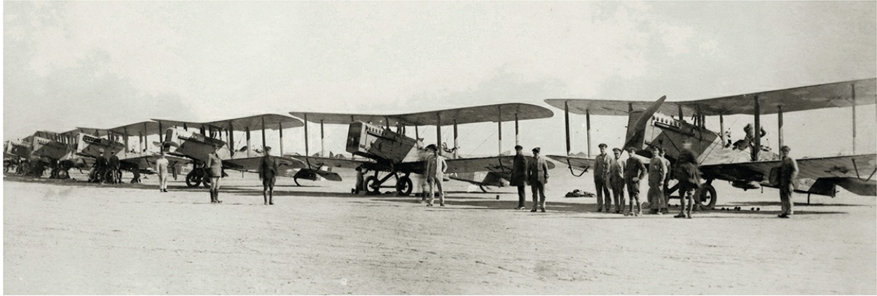
The replacement of the Siddeley Puma engine in the DH9 by a 400hp Liberty engine produced the DH9A – the aeroplane which epitomized the RAF during the 1920s. Known in service as the ‘Nine-Ack’, the DH9A served with squadrons in the UK, Iraq, Palestine, Aden, Egypt and India. These aircraft are from 30 Squadron in Iraq during the late 1920s. (Pitchfork)
