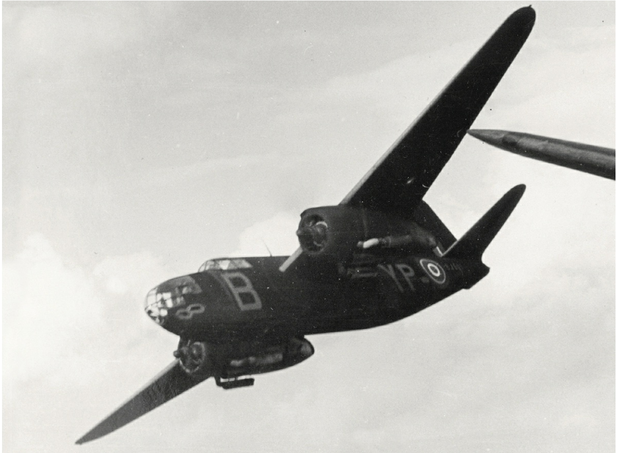
A Douglas Havoc I (also known as the 'Moonfighter') night intruder of 23 Squadron. The aircraft was originally delivered to the RAF as Boston II light bomber. The Havoc was used to patrol over Luftwaffe airfields at night, and attack enemy aircraft as they returned to their home base. (23 Squadron Archive)
