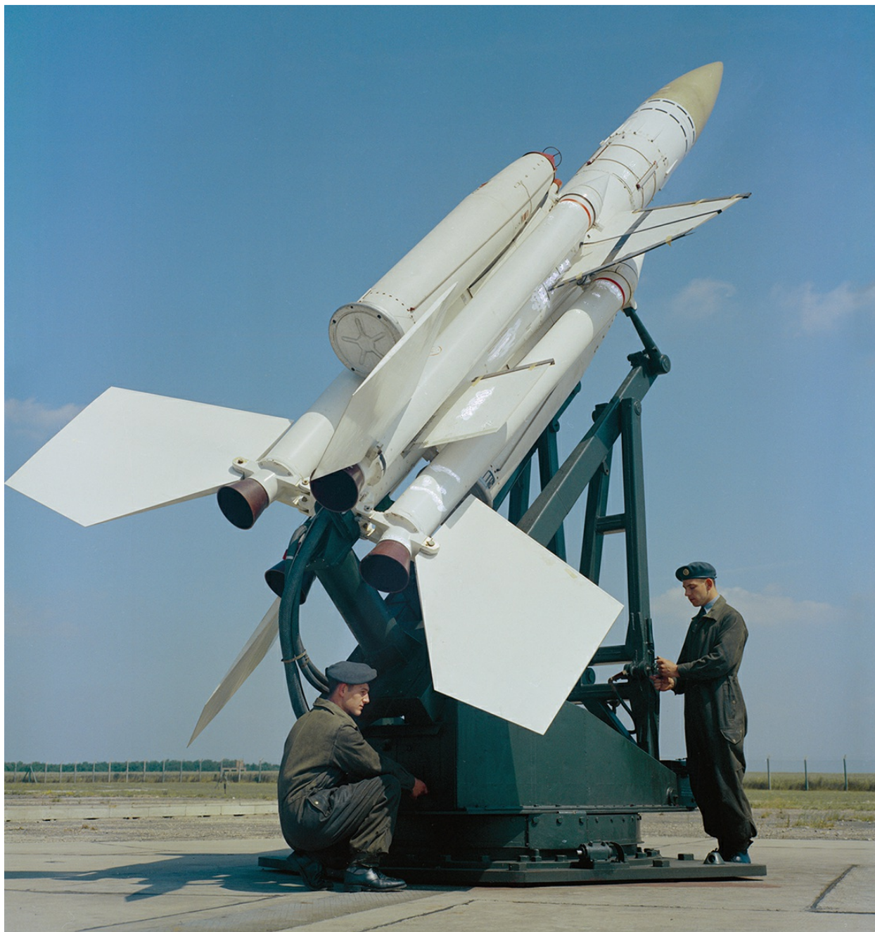
The Bristol Bloodhound Mk1 surface-to-air missile (SAM) equipped ten air defence missile squadrons within Fighter Command for defending V-bomber and Thor bases. The system, which entered service in 1958, could engage targets at altitudes up to 50,000ft. (© IWM RAF-T-2703)
