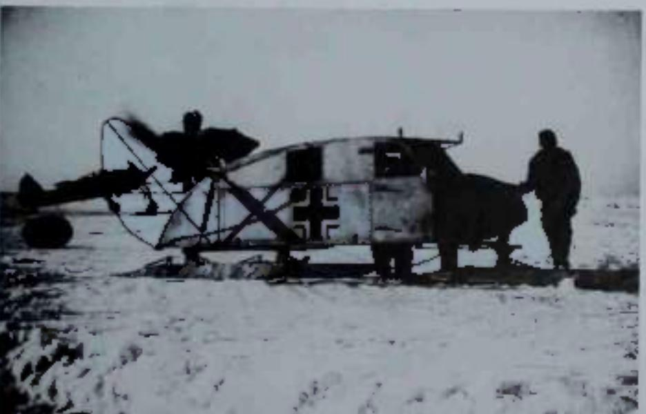
*Bottom: This captured Soviet aero sledge served in a more spartan role with JVJ-JU 51 'Mölders'. The odd-looking craft was powered by a light aircraft engine driving a pusher propeller. It was an original Soviet design, widely used on the Eastern Front. Fitted with armoured plating, these aero sledges spearheaded attacks across enemy expenses; others were used as ambulances or for liaison.*
