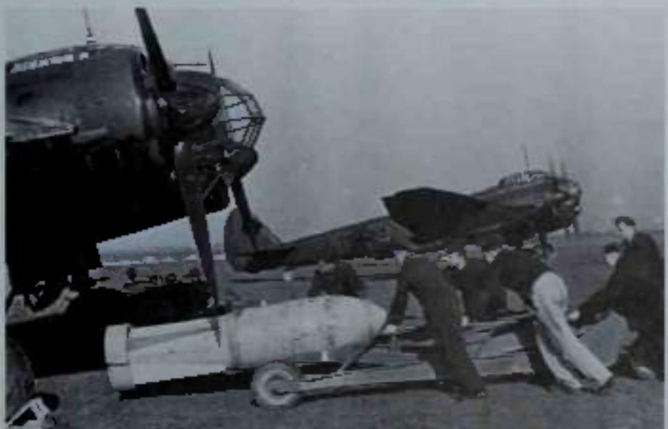
*Bottom: Ju 88A-1s of II/LG 1 are being loaded up with 1000kg (2205lb) SC 1000 bombs carried on external bomb racks. In this case, the night camouflage paint has been used to cover the nationality markings as well.*
