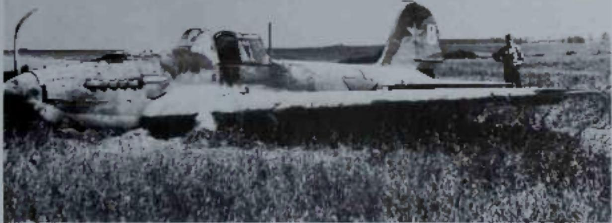
*Top: A closer look at a shot-down Soviet Ilyushin Il-2 ground-attack aircraft. Known to German troops as the "Zementer" (Concreter), it was built around an armoured shell. At times swarms of these machines made life difficult for German airfields, road transport and artillery positions.*
