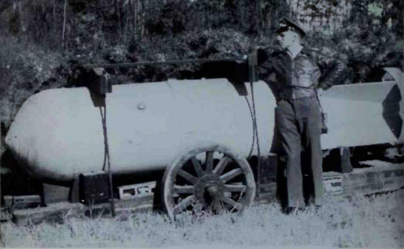
Top: The heaviest bomb used by the Luftwaffe was the 2500kg (5511lb) S.R. 2500 'Max'. Its explosive charge amounted to 1709kg (3748lb). Here is a 'Max' on its special carriage destined for KG 1 'Hindenburg' at Dno in spring 1942.
