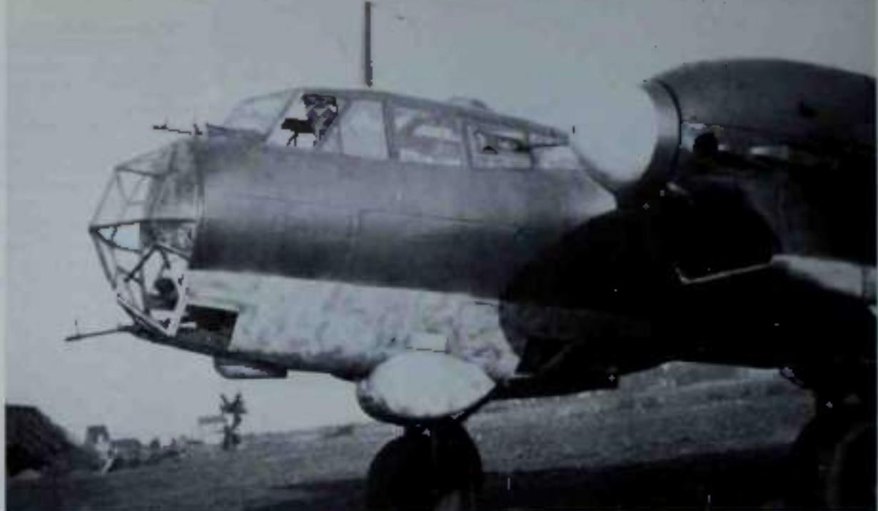
*Top: The Do 215B-4s of 4./Fj. Aufkl.Gr. Ob.d.L. (see Glossary) based at Merseville carried out increasingly more frequent flights over the British Isles; it was important to complete the target reference maps for the forthcoming Operation 'Adler'. The vertical bulge under the forward fuselage of this Do 215B-4 of the above unit contains the Rb. 70 x 30 automatic aerial camera.*
