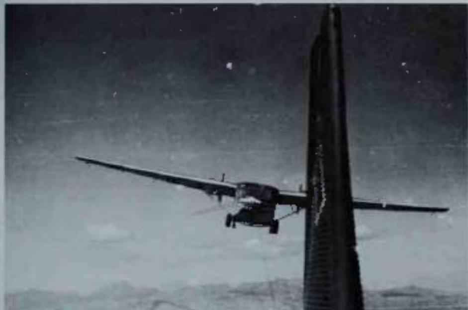
Centre: The severe losses of German and Italian shipping led to a change in tactics and from early 1942 on increasing use was made of air supply of Axis forces in North Africa. Shown here is a Go 242 cargo glider in tow behind a Ju 52/3m. [The main reason for these shipping losses was information obtained via ULTRA at Bletchley Park; by mid-1941 the British were able to read most of the secret Luftwaffe 'Enigma' machine-coded messages dealing with supplies and the deployment of units. Tr]
