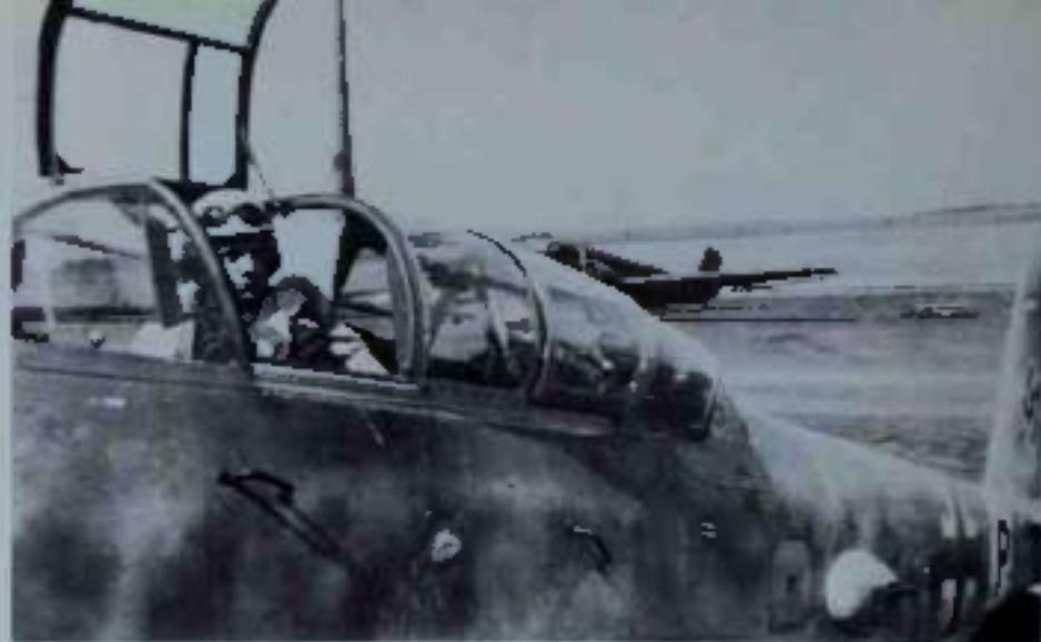
*Centre: Lt Peter Bauer of 3./JG 76 in a Me 410B 2/U2/H5. The standard armament of this 'Zerstörer' version consisted of eight 20mm MG 151/20 cannon and two 7.92mm MG 17 machine guns. Under ideal conditions, this concentrated firepower could literally 'gut' a four-engined bomber to bits.*
