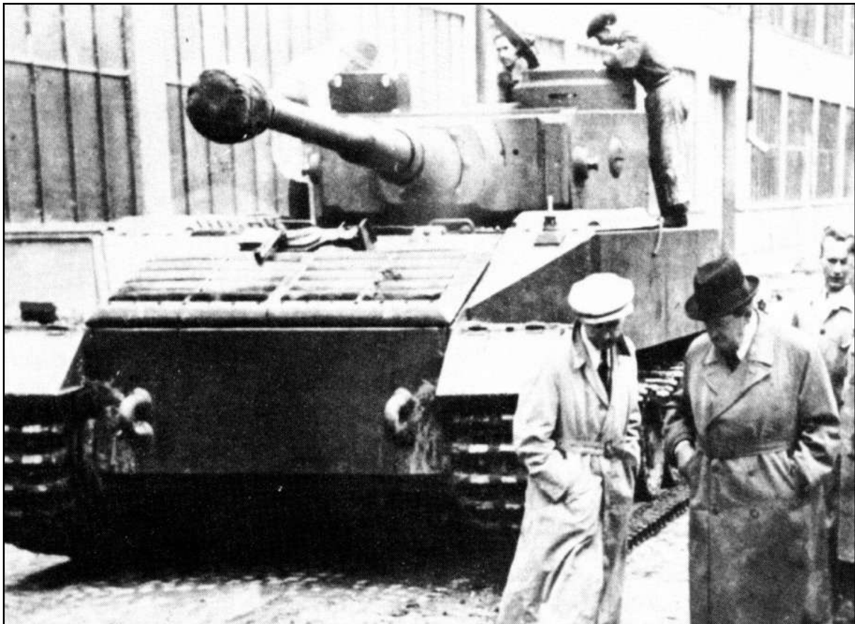
At St Valentin Porsche (right) conferred with colleagues next to a Tiger (P) with its 88mm gun pointing rearwards. Extensive venting in its rear deck was needed to cool its engines and electrical machinery.
