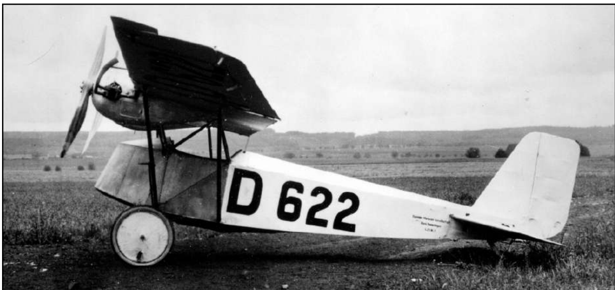
In 1925 Daimler's Sindelfingen Works introduced this Klemm-designed parasol monoplane, the L 21. Equipped with two F7502 twins, a sister L 21 to this aeroplane won its 40bhp class in 1925's Round-Germany Competition.
