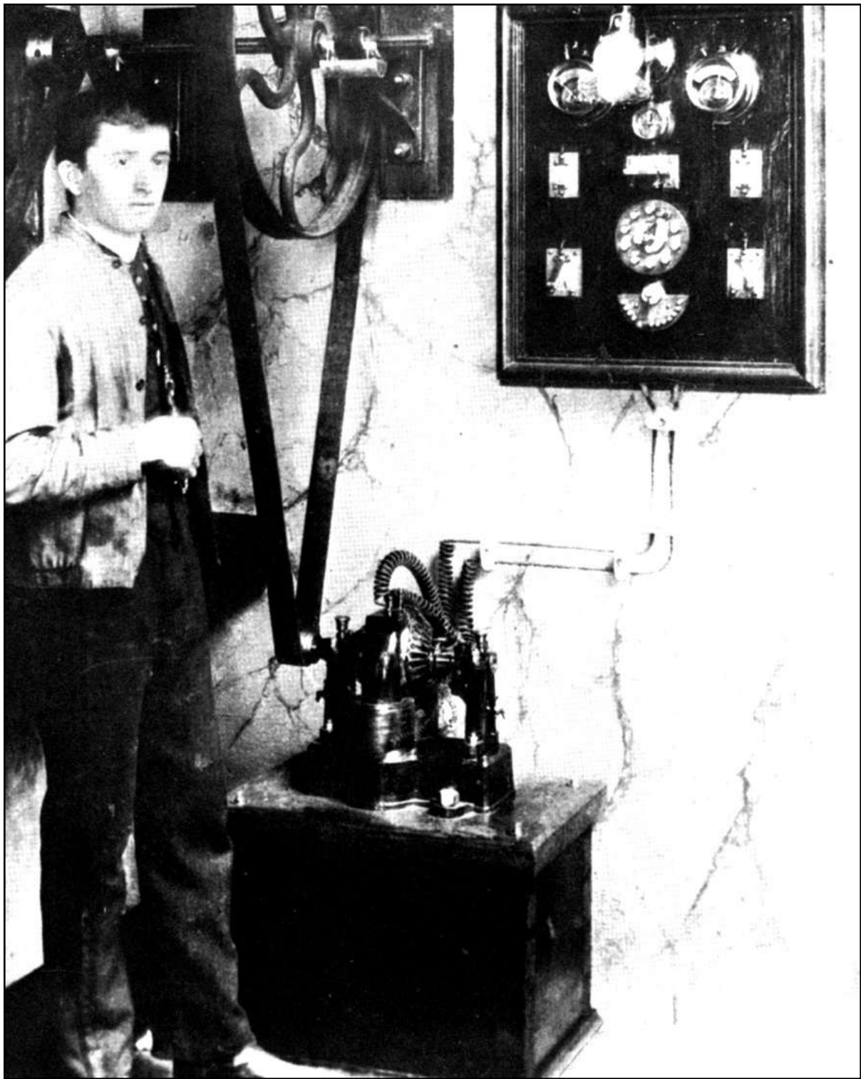
By the age of 13 Ferdinand Porsche had electrified both his home and his family's workshop in Maffersdorf. A shaft from the workshop's machinery drove a high-speed dynamo, its output controlled from a master board.
