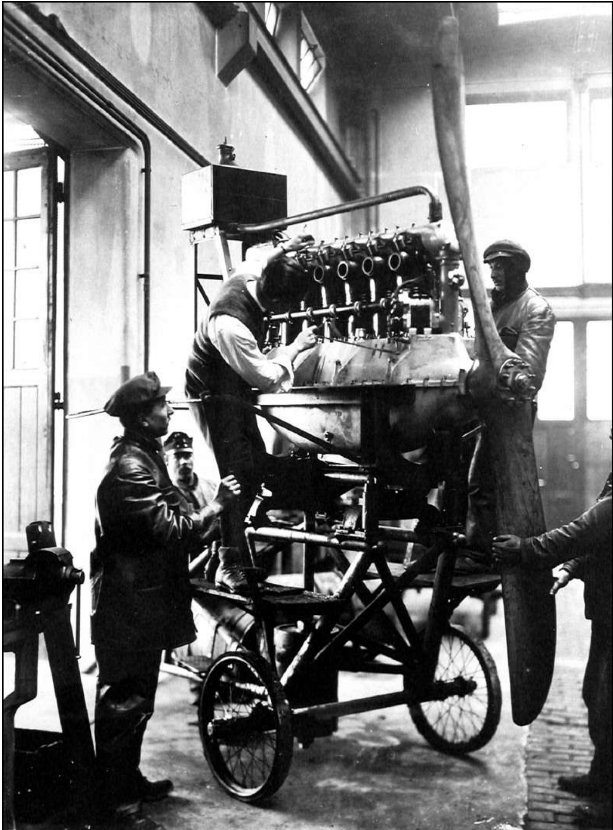
Introduced in 1915, Austro Daimler's 160hp six was a mainstay of the dual monarchy's aeronautic arm. Ferdinand Porsche climbed on the cart transporting one to a test bench to check its overhead-cam valve gear.
