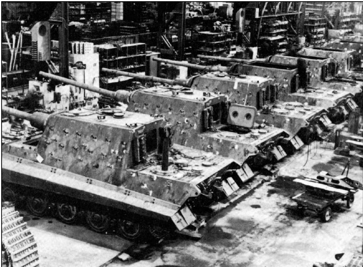
Although these are Tiger (H)-based tank destroyers being built at St Valentin, two with the same superstructure were built on Tiger (P) chassis. They carried long-range 128mm cannon.
