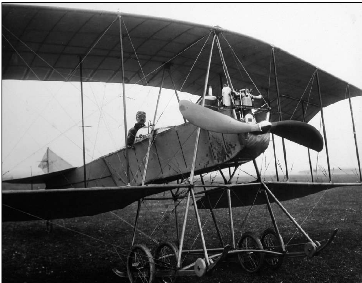
The handsome biplane of Austrian pioneer Adolf Warchalowski gained improved performance with the installation of an Aëro-Daimler four in 1910. Here in 1911 it was piloted by Captain Hans Umlauff von Frankwell.
