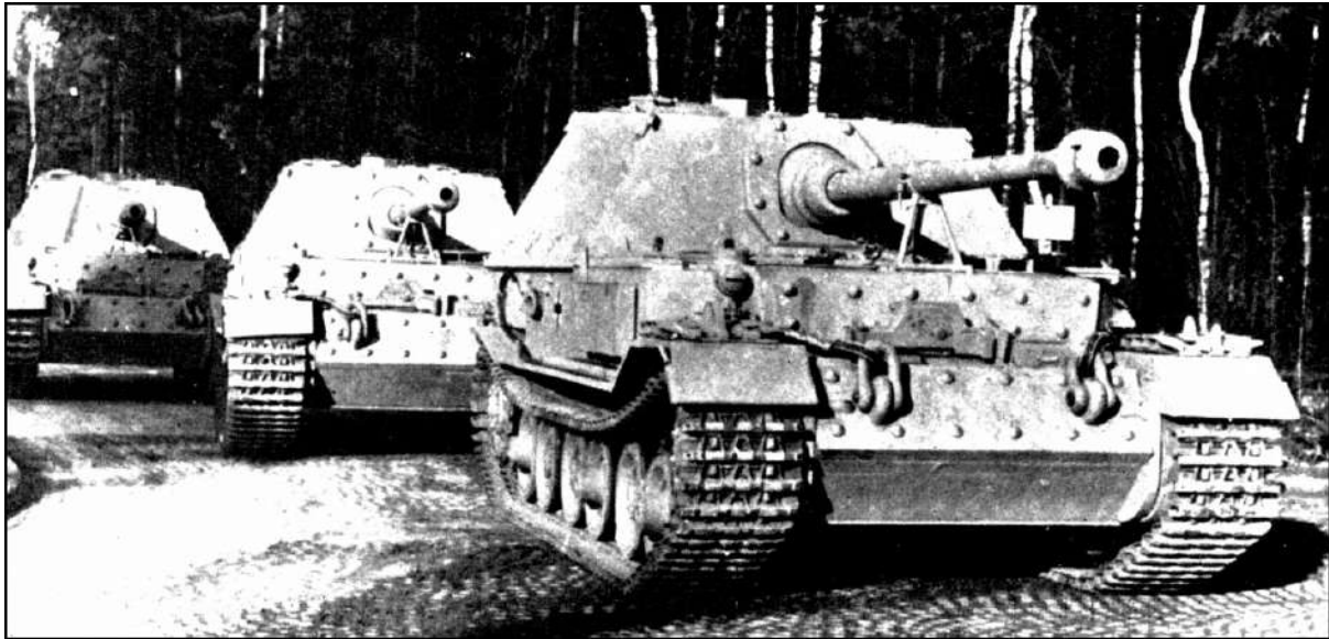
Three fresh Ferdinands showed the extra frontal plating that gave them 200mm armour. Intended as long-range assault guns operating from the rear of an advance, they were not equipped with defensive machine guns.
