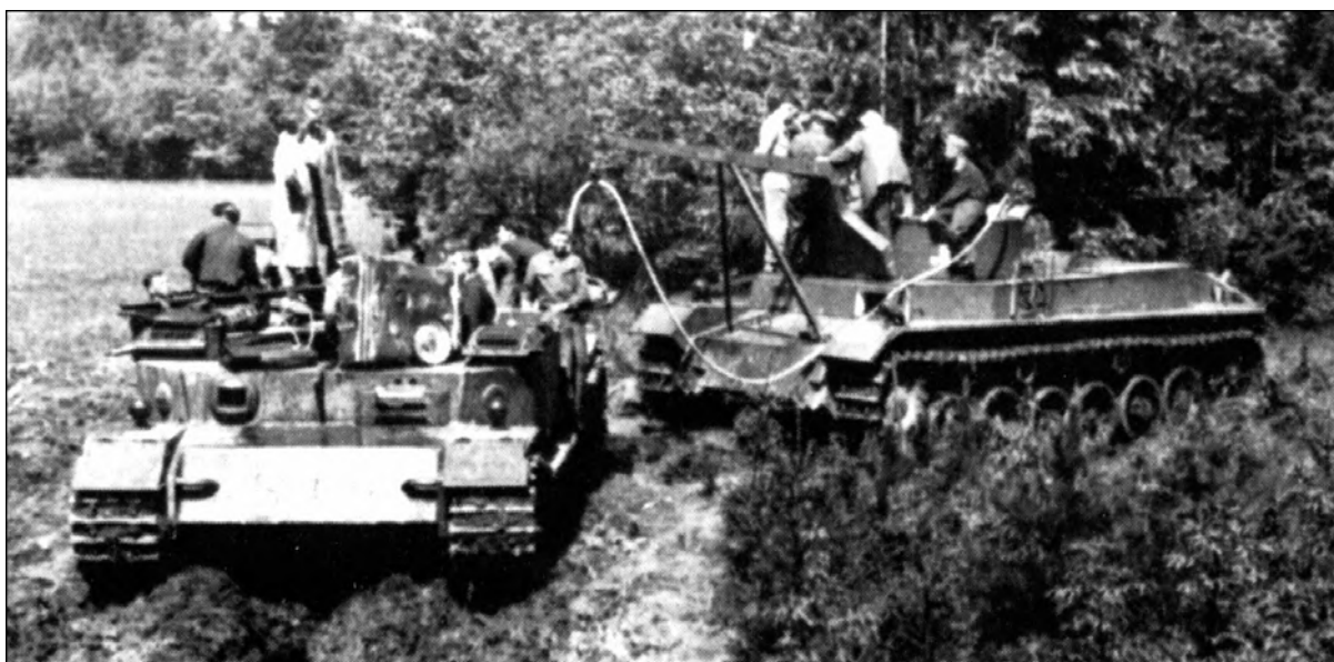
During some trials of the Tiger (P), whose wider tracks are evident, the Type 100 (right) supplied power through cables from its generators. Electrical development was overseen by engineer Otto Zadnik.
