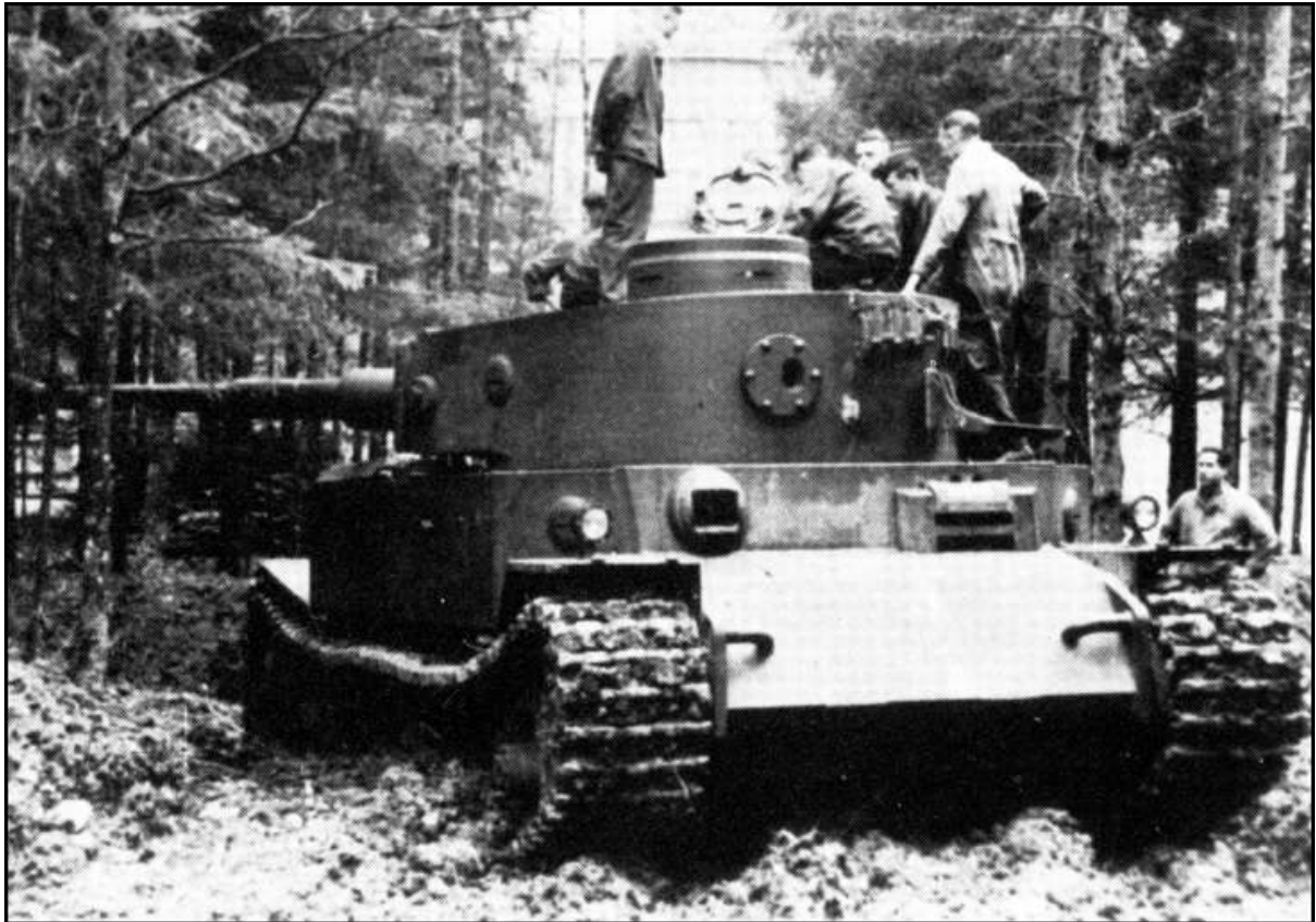
Viewed from its front, the Tiger (P) manifested its 100mm armour, viewport for the driver and ball pivot for a machine gun. Krupp built its electrically traversed turret to Porsche's design.
