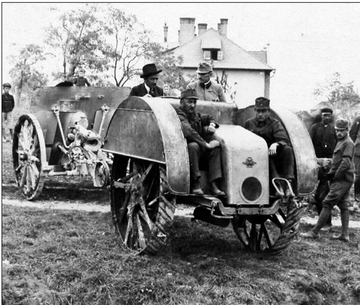
In its developed form the versatile Austro Daimler KP I Pferd was steered at the coupling between the power unit and its cargo, as Ferdinand Porsche personally tested and demonstrated. It also had many post-war applications.
