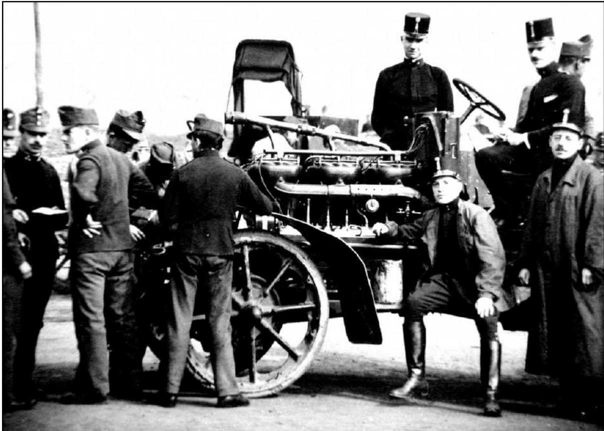
By 1910 troops in the field were getting to know the intricacies of the four-wheel-driven M 08 tug, including its impressive 13.9-litre six-cylinder engine developing 80hp.
