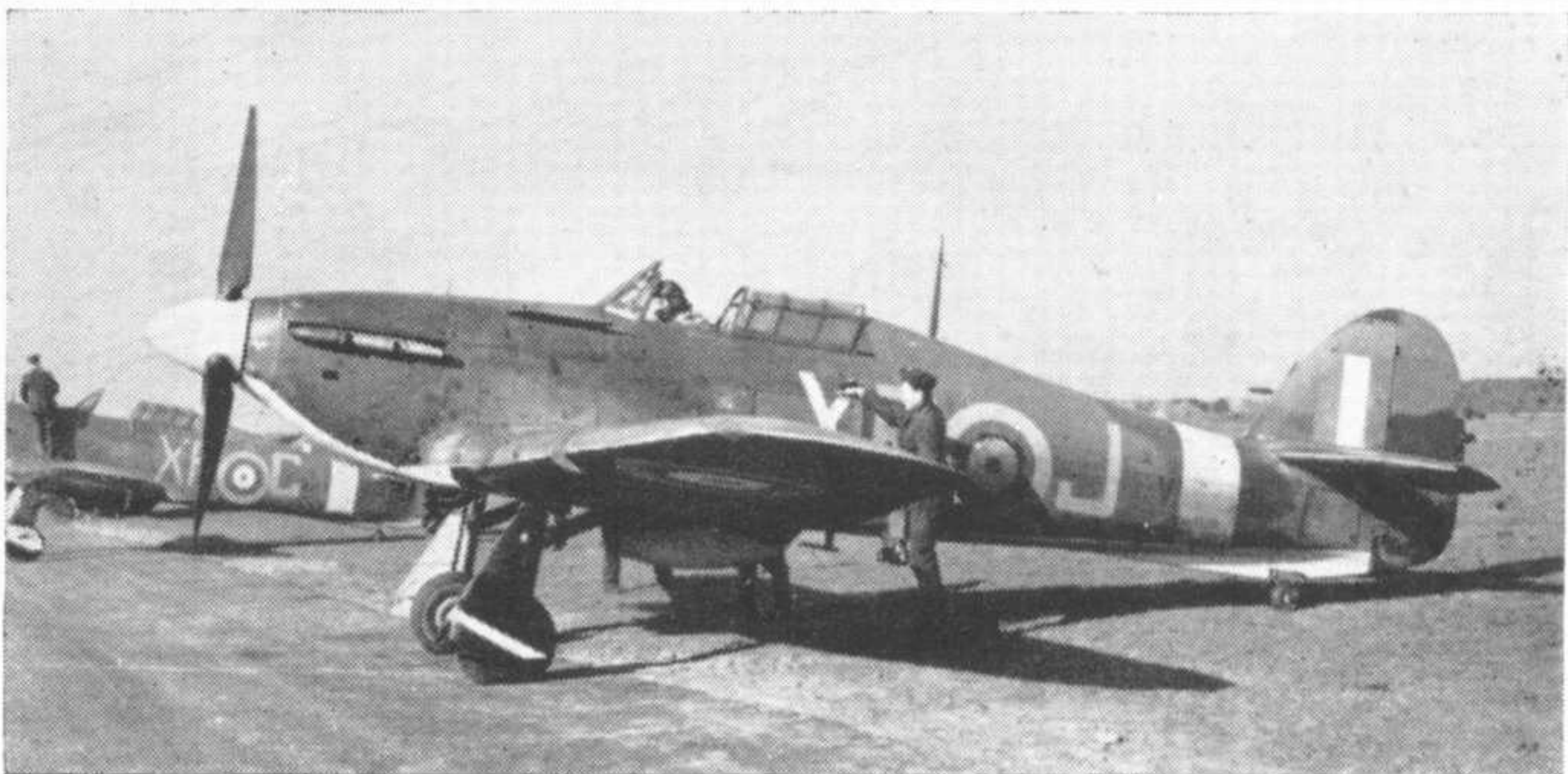
The Hawker Hurricane brought 300 m.p.h. speeds and an eight-gun armament to R.A.F. Fighter Command, and was numerically the most important fighter at the beginning of the war. [Imperial War Museum]
