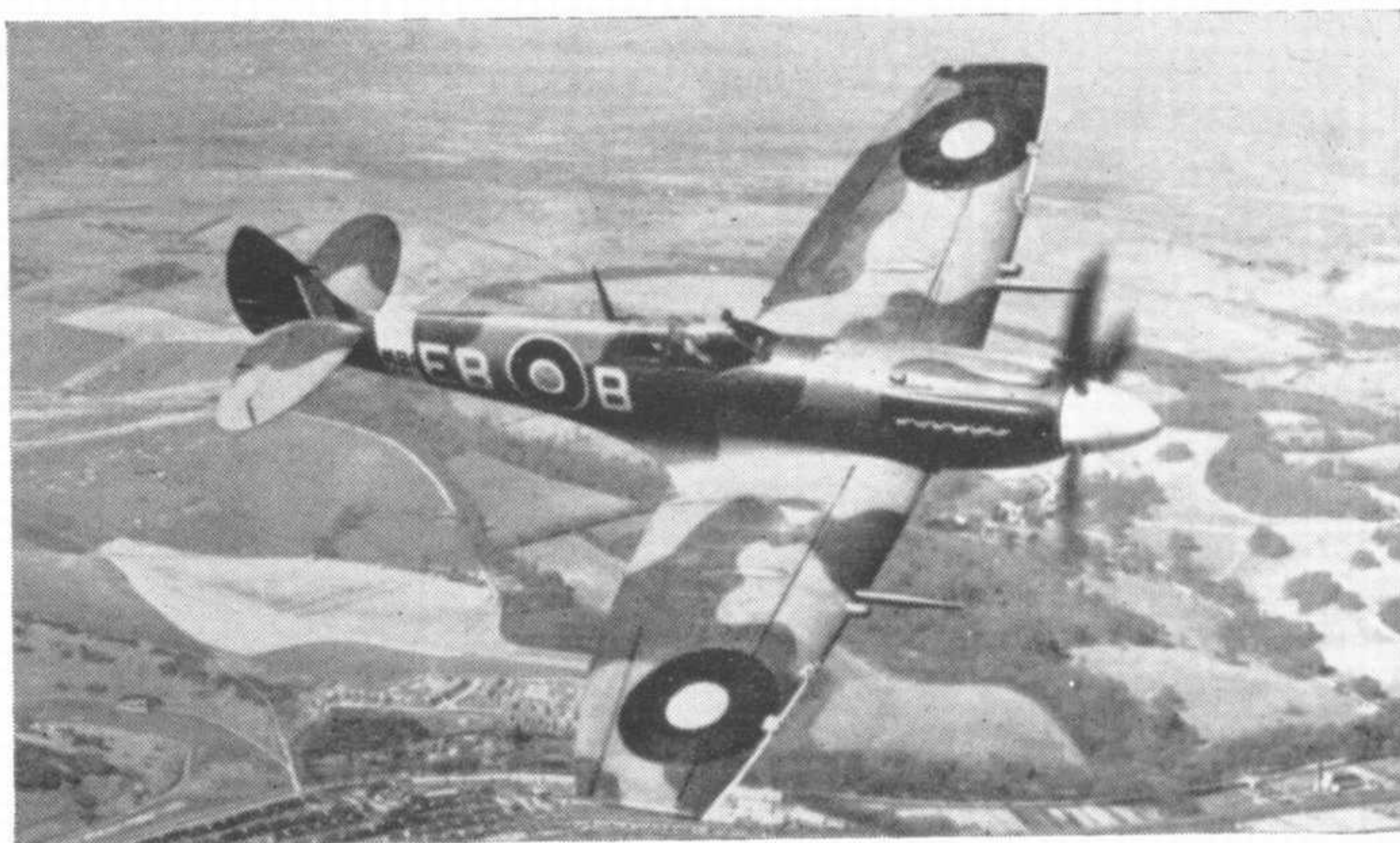
The Supermarine Spitfire remained in production and service from beginning to end of the Second World War, and was subject to extensive development. Above is a Griffon-engined Mk. XII with clipped wings for low-level fighting. [Imperial War Museum]
