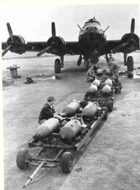
ABOVE: 500lb GP bombs being loaded into a B-17F. This was the most widely used bomb by the Eighth Air Force, with 1,365,387 dropped on Germany and occupied Europe DONALD NIJBOER
