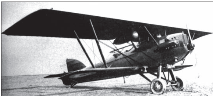
A Paraguayan Air Arm Potez 25A.2 fitted with the reserve fuel tanks. (Musée de l'Air)
