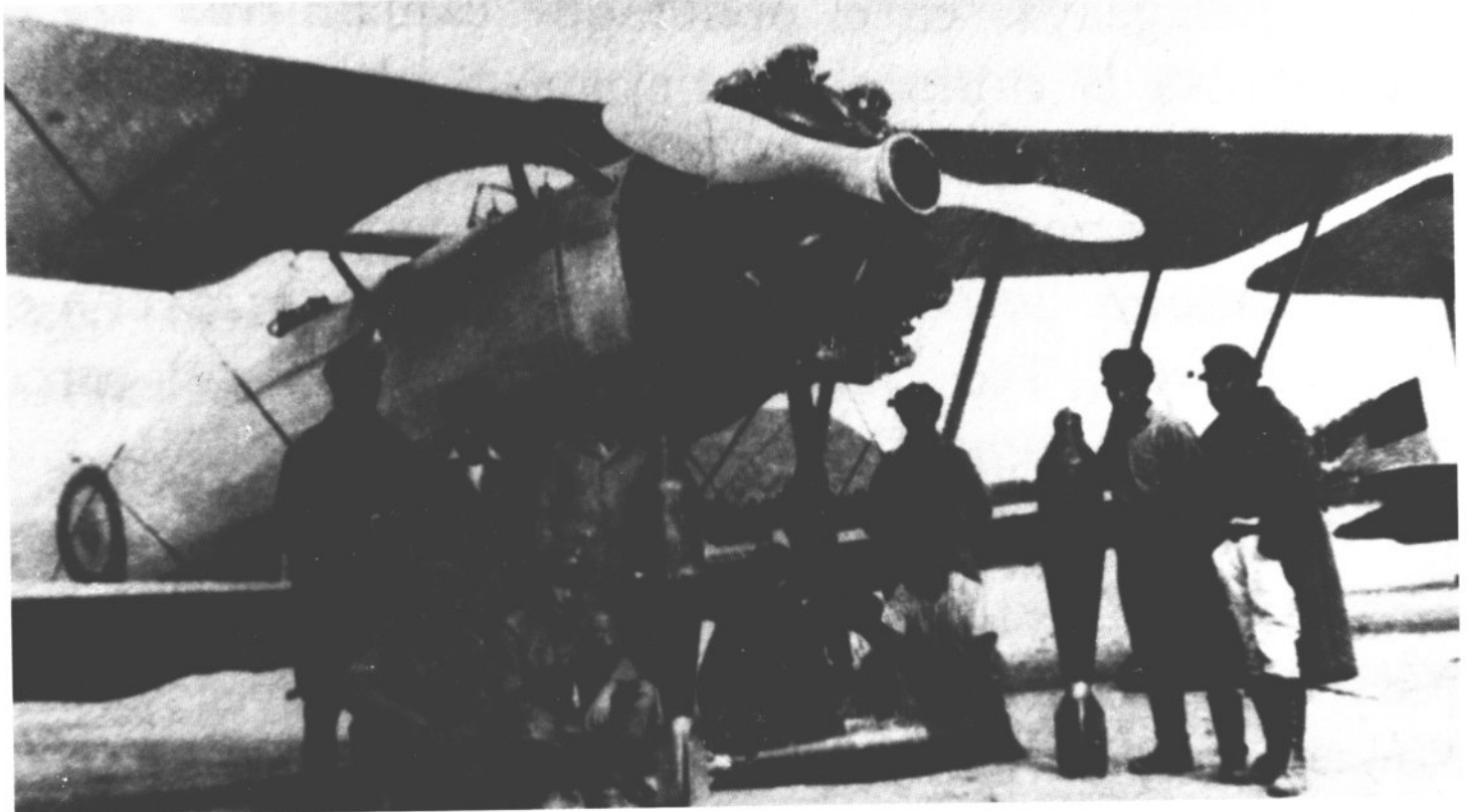
Bolivian crews in the area of operations before a pair of "Vespa IIIs" and displaying two of the largest caliber bombs used during the war, one of which could be carried at a time by a "Vespa" under the mid-fuselage (via Georg von Roitberg).
