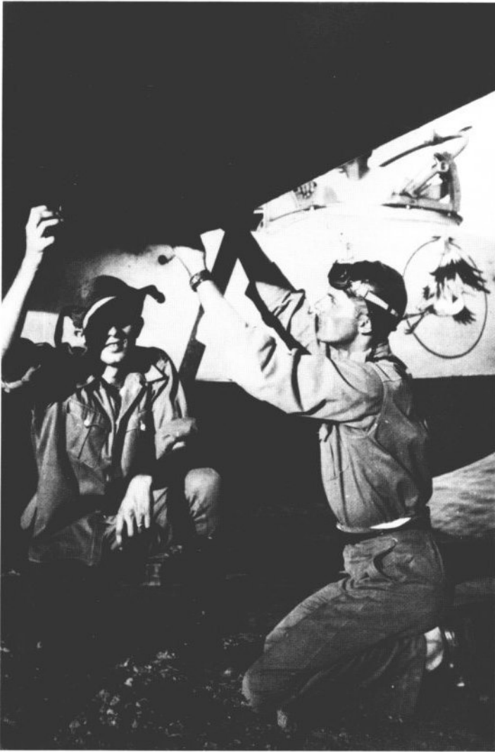
Ground crews of the Paraguayan Navy inspect the underwing starboard bomb rack of a Macchi M.18A.R. at Bahía Negra in 1934. The special insignia carried on both M.18s is visible in the background (Aviación Naval Paraguaya).
