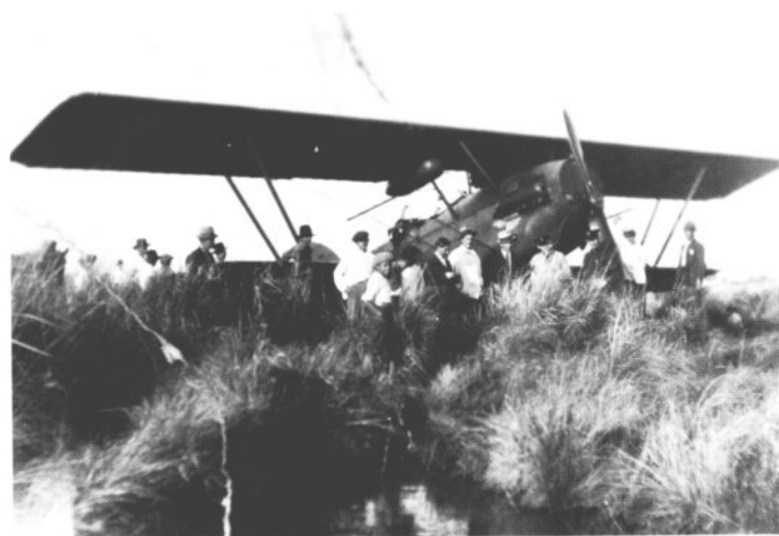
An unidentified Paraguayan Potez 25 at the Paraguayan Isla Poí aerodrome, showing the extremely rugged conditions there and also the rarely seen auxiliary fuel tanks under the upper inboard wing panels (Archivo Cnel. Av. (S.R). A. Pasmor).
