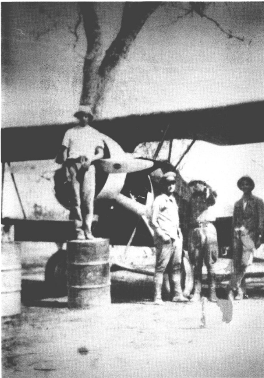
In this 1933 photo of the single Paraguayan Consolidated Model 21-C (frequently cited in error as a "PT-11") the fuselage of the aircraft appears to have been painted a dark color, although the cowl ring and underside are light. It is seen here at Isla Poí. (Archivo Cnel. Av. (R.S.) A. Pasmor).
