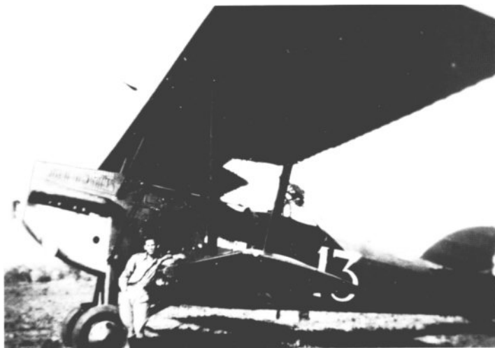
The rather beefy profile of the Potez 25 T.O.E., compared to the standard Potez 25 A2, is evident in this side view of s/n 13, which appears to have had a name painted on the mid-fuselage (Archivo Cnel Av. (S.R). Agustín Pasmor).
