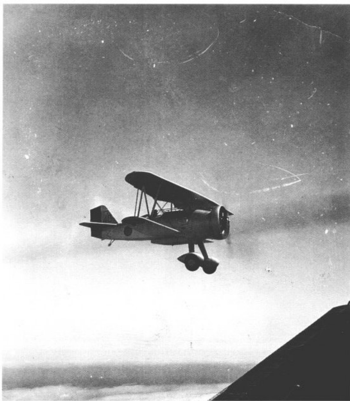
The beautiful Curtiss "Hawk II" fighter-bomber, although acquired in comparatively small lots by Bolivia, etched an indelible legacy in the Chaco air war out of all proportion to its numbers. Here, s/n 40, the fourth example received circa August 1933, is shown in full markings in flight over the Chaco, complete with belly auxiliary slip fuel tank (Ramiro Molina Alanes).
