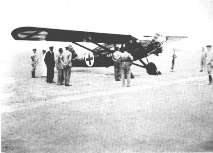
Paraguay also had air transport and ambulance needs, but did not enjoy the luxury of an established, well-equipped internal airline to nationalize. Instead, agents acquired used but adequate transports where they could. This Travel Air Model 6000, serialied T-9 and named "Nanawa," still bears its former U.S. airline name "Boston," besides full Paraguayan ambulance and national markings in this 1933 photo at Ñu-Guazu. (Archivo Cnel. Av. (R.S). A. Pasmor).
